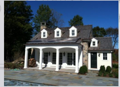
Cottage with Solar array on roof
